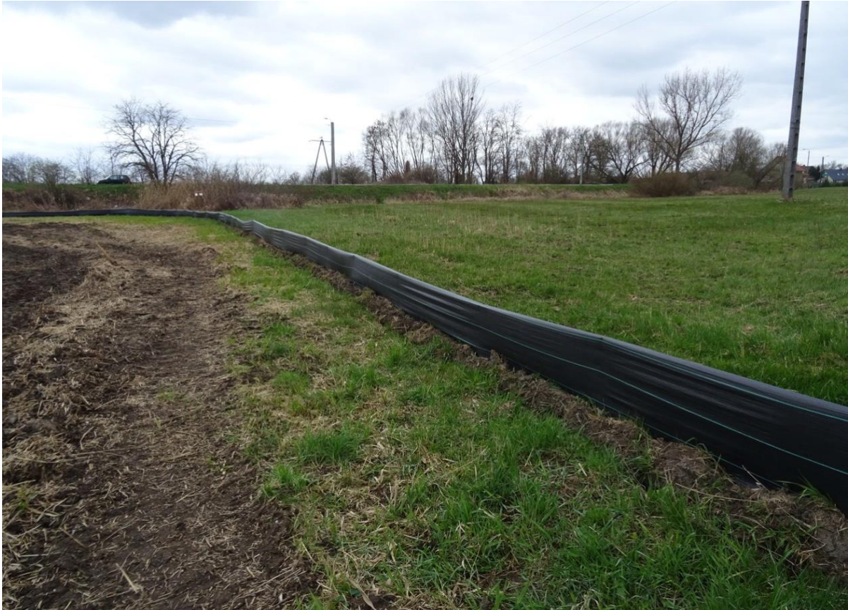
Photo 5. Example of the Use of Herpetological Fences at the Project Site, Also Serving as Barriers for the Protection of Natural Habitats
