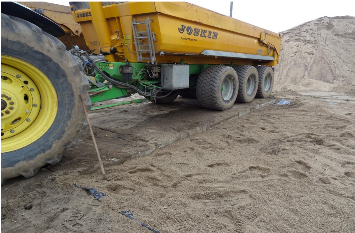
Photo 6. Hardening of Machine Parking Areas Using Foil and Plates
