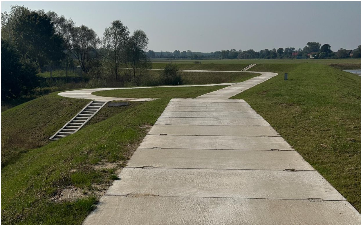
Photo 12. Grass Growth on the Seeded Slopes of Embankment No. VI
